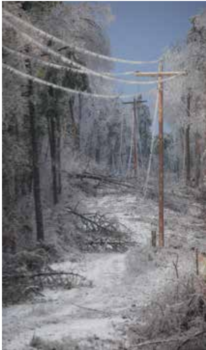
As little as a quarter inch of ice is enough to bring down power lines.
